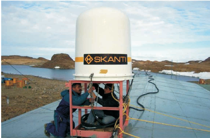
Fig. 2: INMARSAT terminal being maintained by DEAL team
