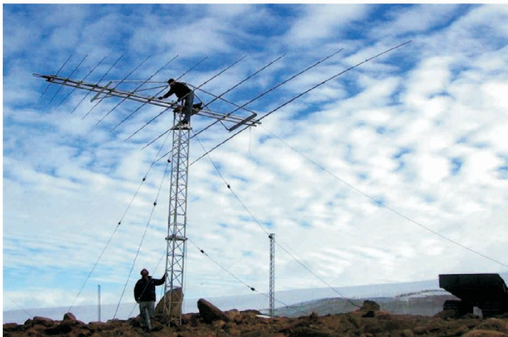
Fig. 3: DEAL team repairing HF antenna after blizzard
