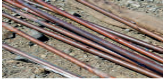
“Damaged pipes of the defunct water duct line”
