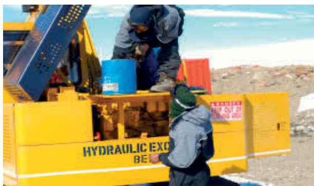
“Commissioning of a defunct Hydraulic Excavator”
