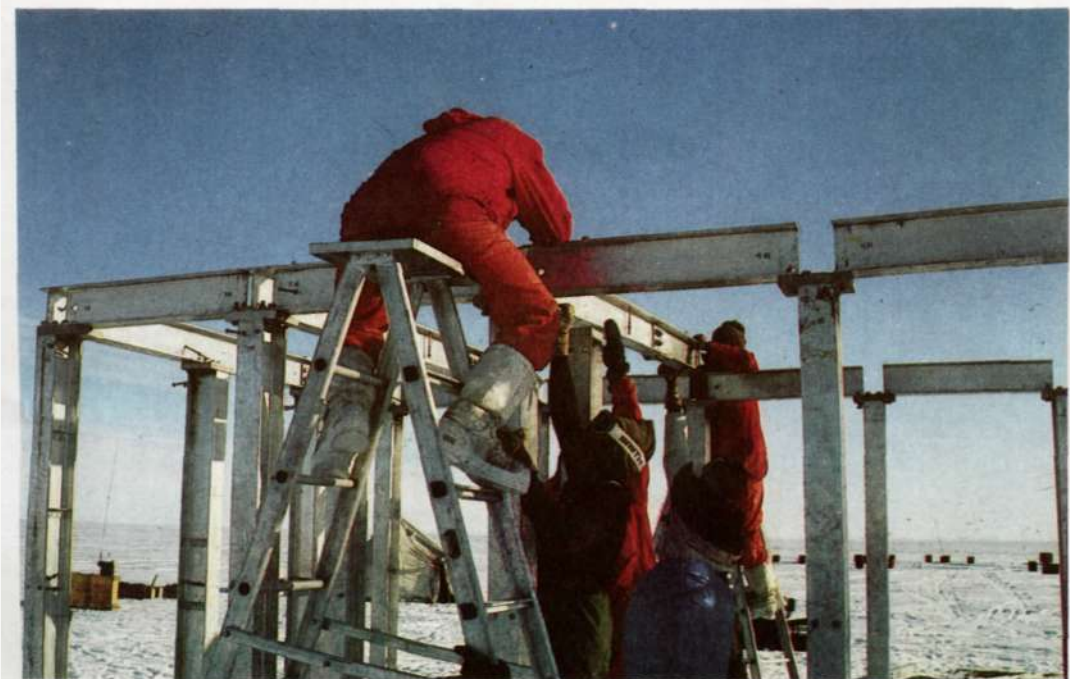
Construction work of a barrack commences in Antarctica.
