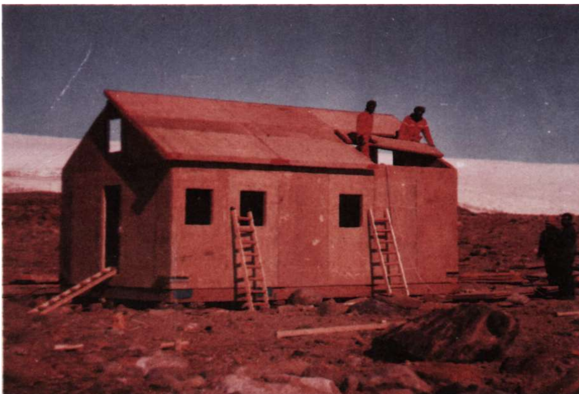
Fig. 7. Cottages of Maitree station under construction (Photograph: B.B. Bhattacharya)
