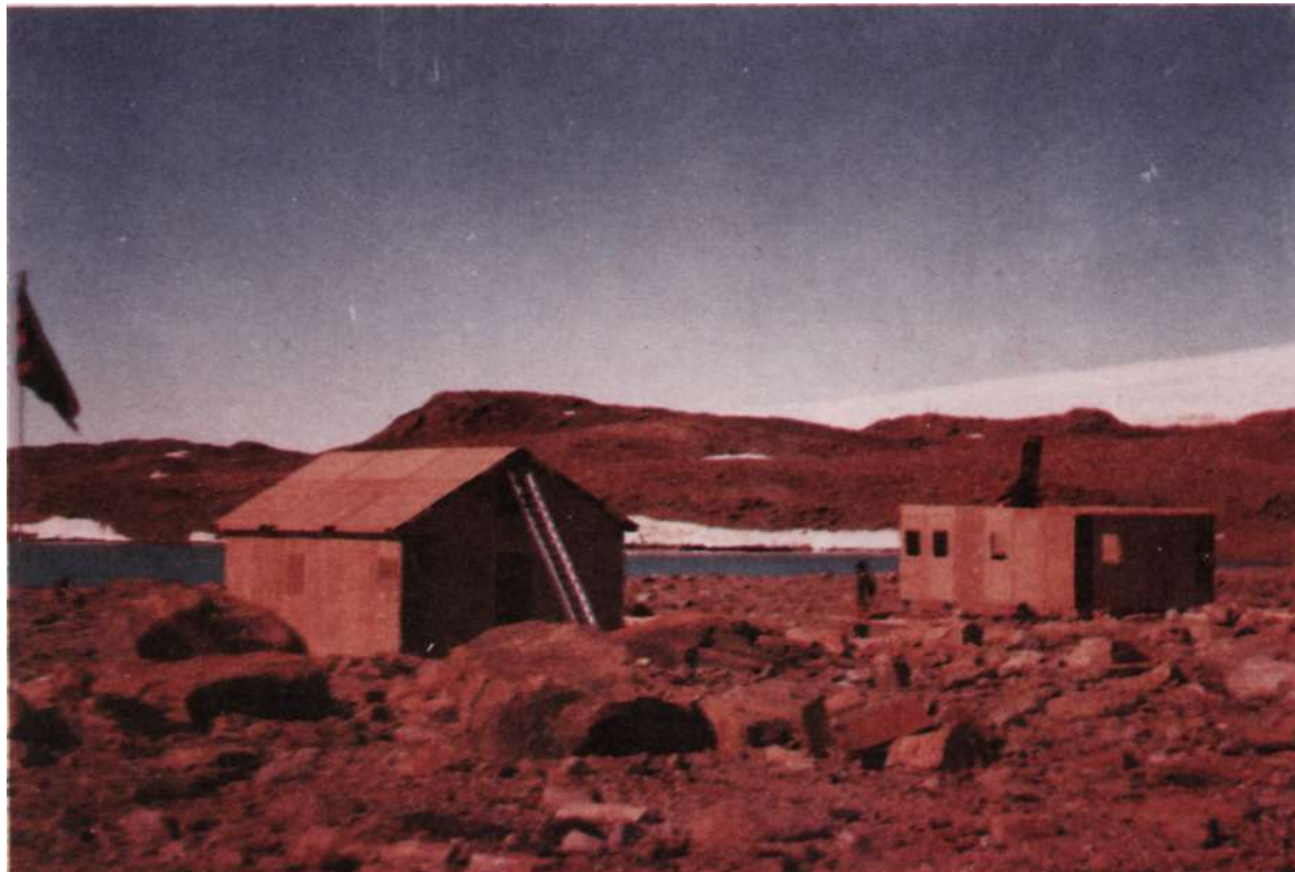
Fig. 8. Maitree station more than fifty percent complete (Photograph: B.B. Bhattacharya)
