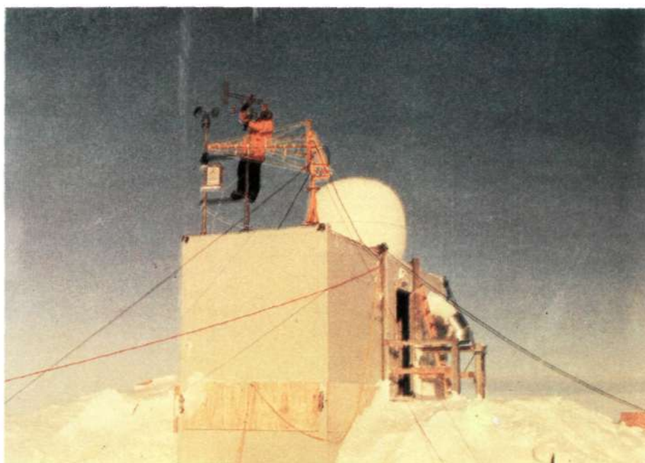
Fig. 2. Installation of the data collection platform (DCP) atop hangar garage at Dakshin Gangotri station
