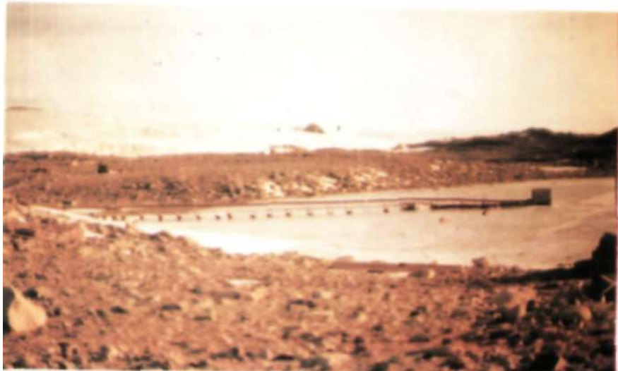
Fig.8. Drinking water pipeline at Maitri.
