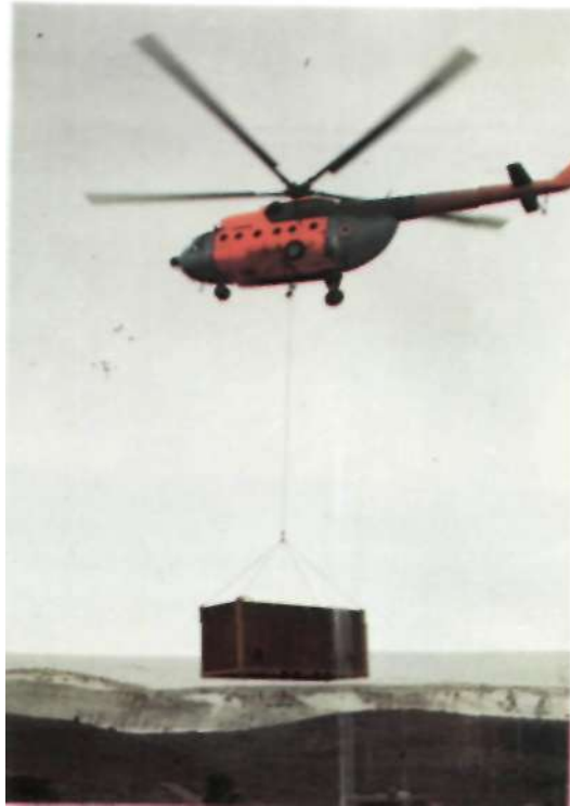
Fig.9. Placing a container at Maitri.
