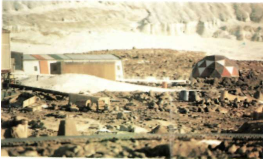
Fig.5. The generator accommodation, greenhouse dome and bio- digester at Maitri.
