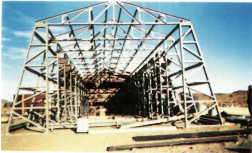
Fig. 10. Generator accommodation under construction.
