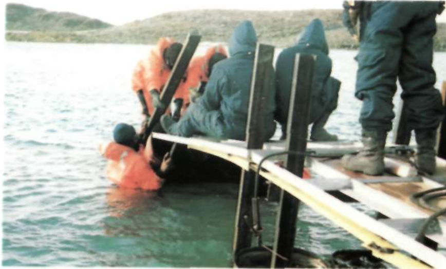
Fig.7. Strengthening the pump house foundation.
