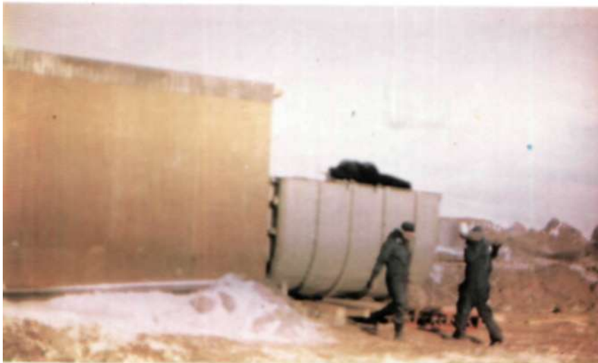
Fig.6. Installing the B3 Klargester (bio-digester).
