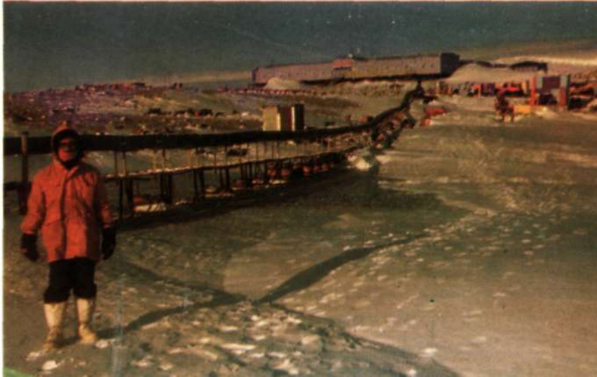
Fig. 2. Water-supply pipe line between the Pump House and Maitri station.
