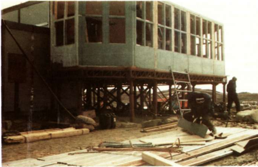
Fig. 5. GH under construction.
