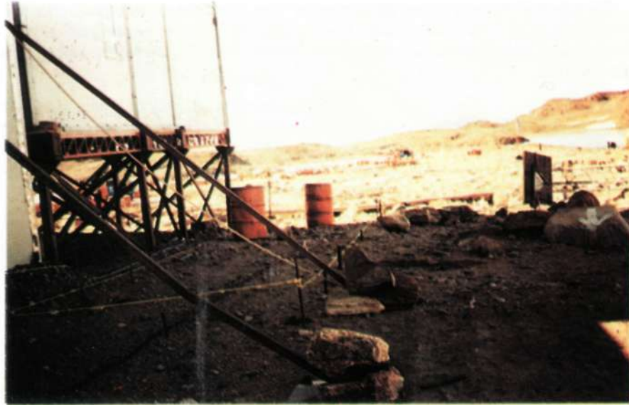
Fig. 3. Marking of site for foundation work of GH.
