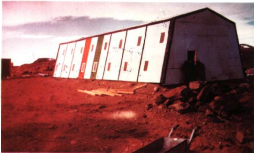
Fig. 1. Generating set accommodation.
