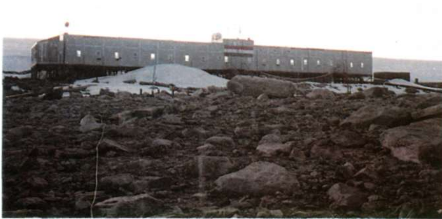
5. Maitri building during a winter night
