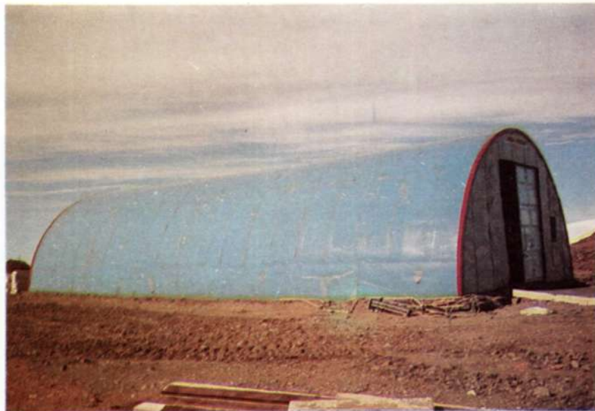
4. SHELTER AFTER ROOFING
