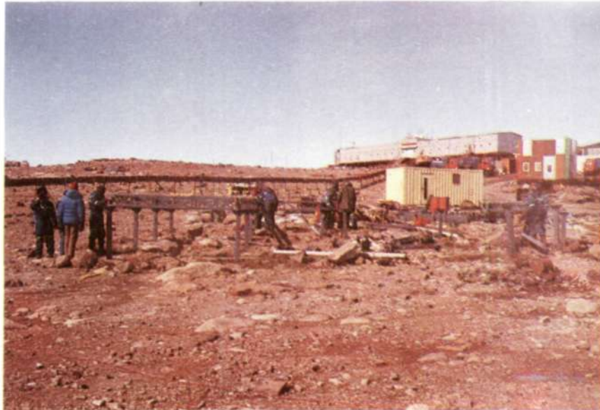
7. ERECTION OF FOUNDATION STRUCTURE
