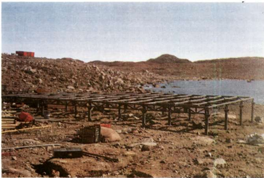
8. ERECTION OF FOUNDATION STRUCTURE
