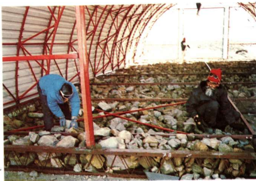
6. PITCHING OF FOUNDATION STONES
