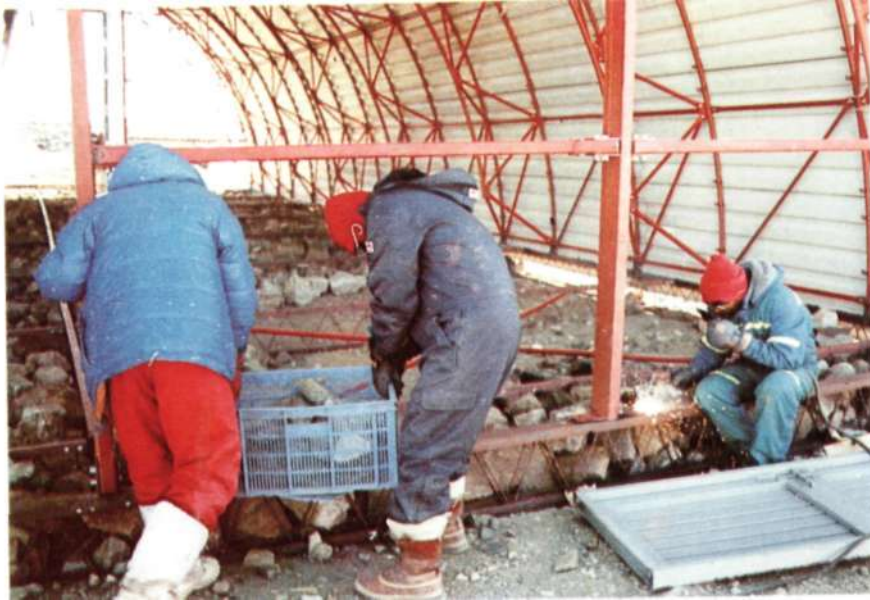
5. WELDING AND FILLING OF FOUNDATION
