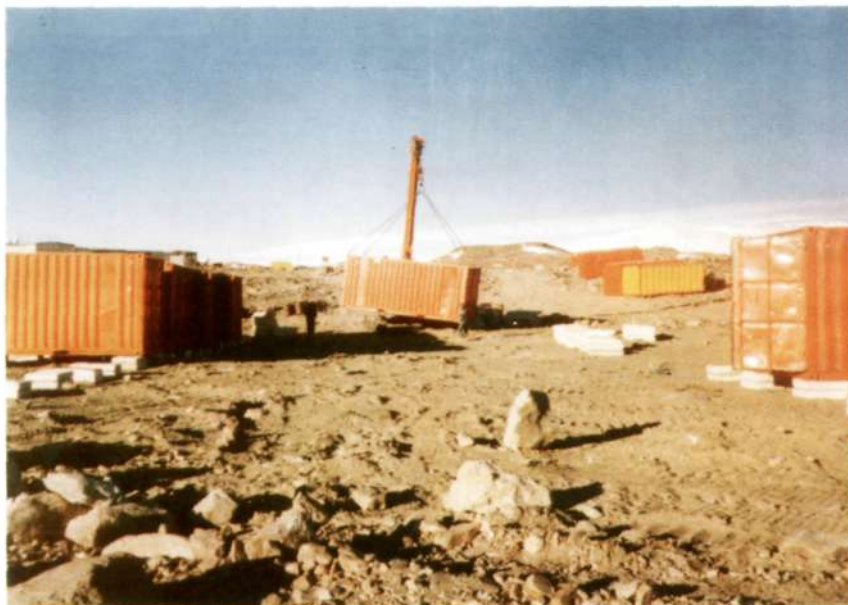
Container complex in the making at Maitri Station (April 1997)
