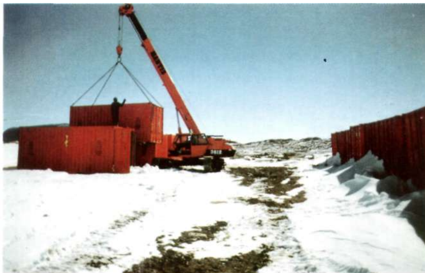
Container complex with Snow accumulation (Oct 1997)
