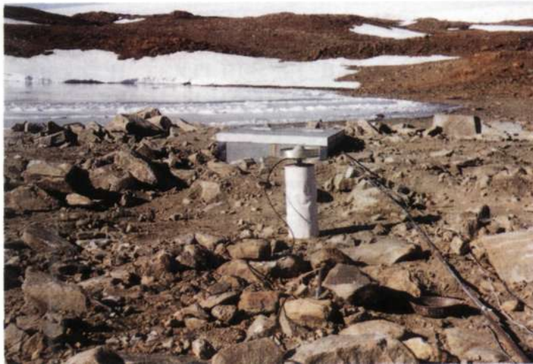
Figl. GPS Choke Ring Antenna mounted on a Permanent Concrete Pillar.
