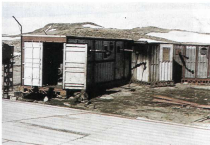
GENERATOR HUT COMPLEX - MAITRI
