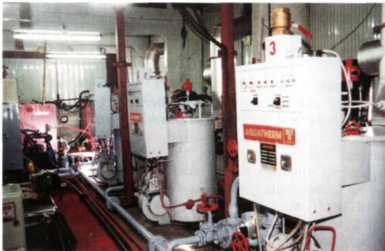
Renovated boiler room
