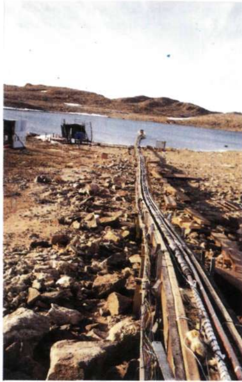
Installation of new pipe line with electrical trace heating
