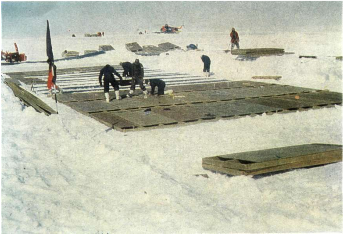
Fig. 8. Foundation of Dakshin Gangotri station
