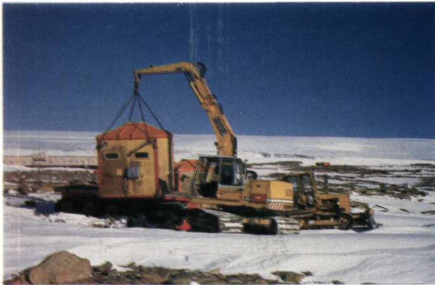
Re-location of toilet modules without dismantling; apart of environ-clean up.
