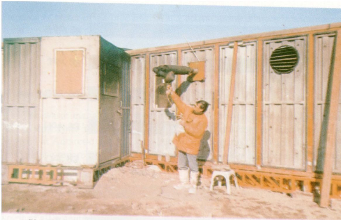
Plate 1: Collection of exhaust gases from source at Aditya Generator Hut
