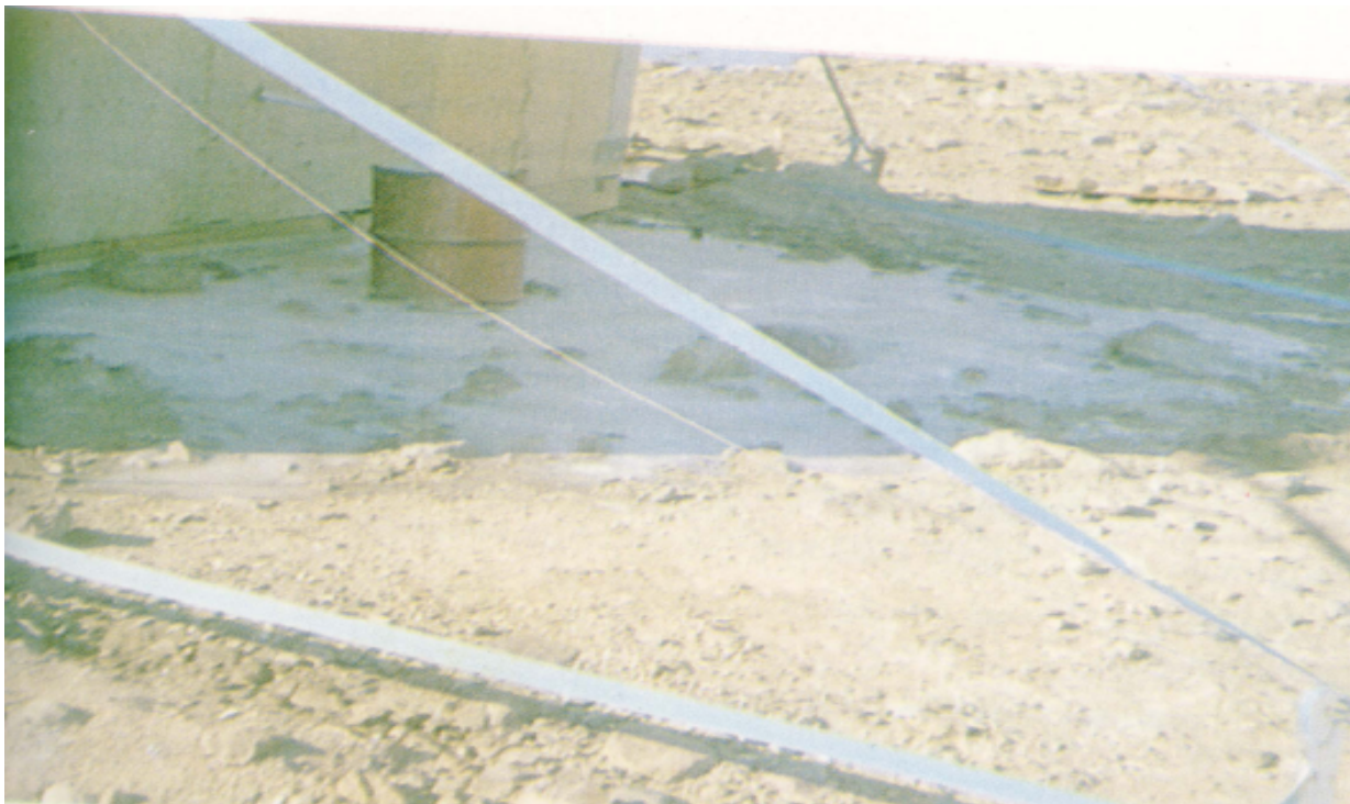
Plate 2: Rubber strips tied with the summer huts generate noise time at wind and cause disturbed sleep in night
