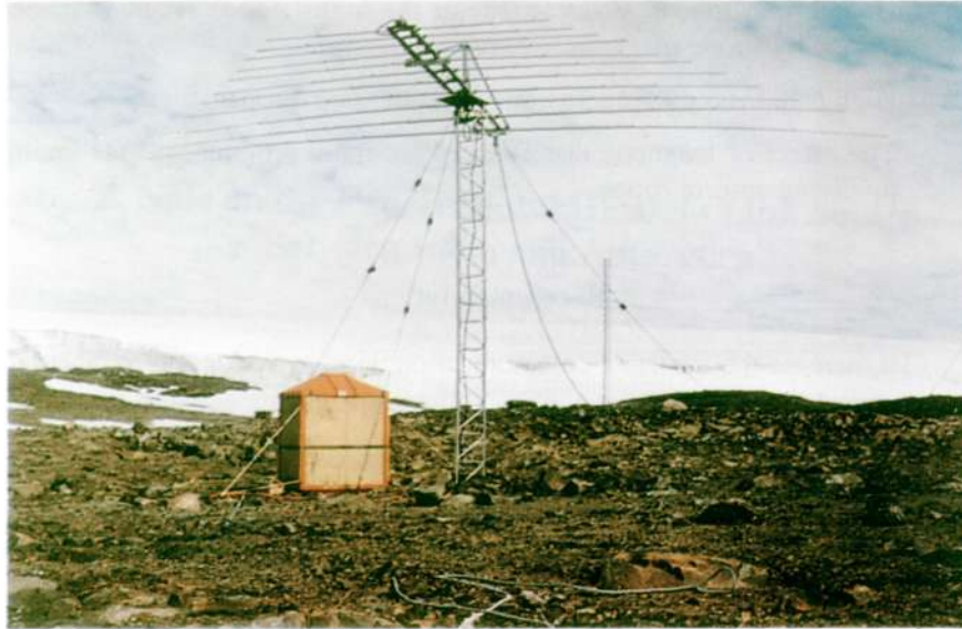
Fig 2 : A compact HF Log Periodic Antenna (LPA) installed at Maitri.
