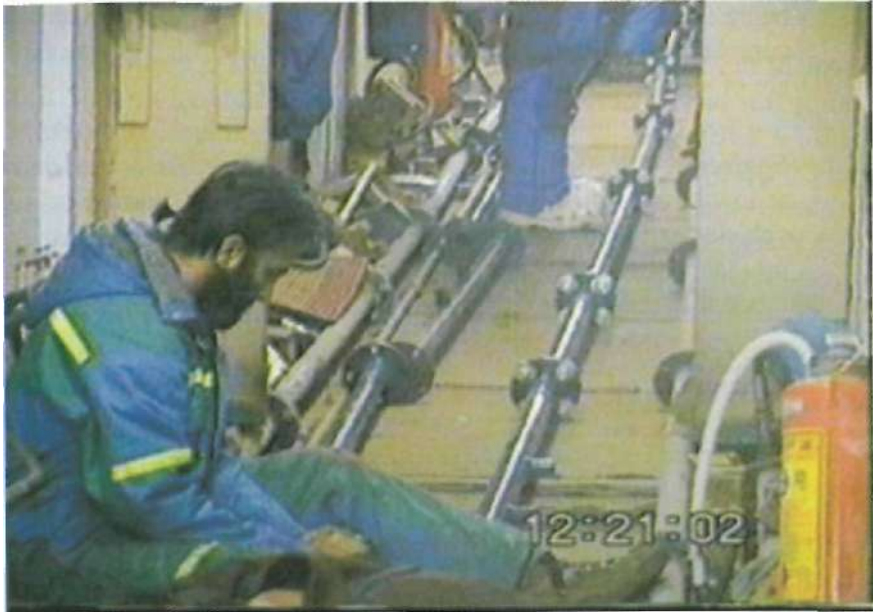
Fig. 6: Hot water pipeline being replaced.
