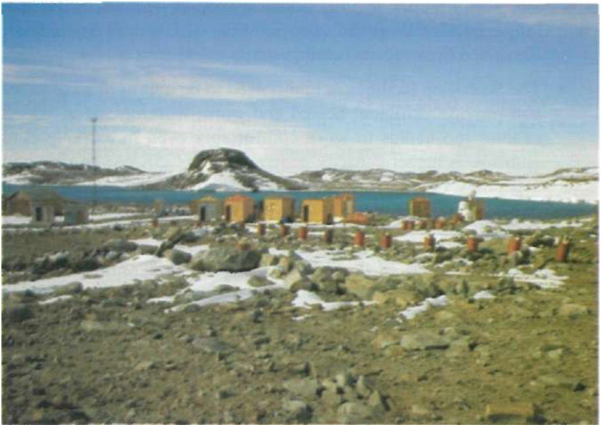
Fig. 9: A View of summer hut area.
