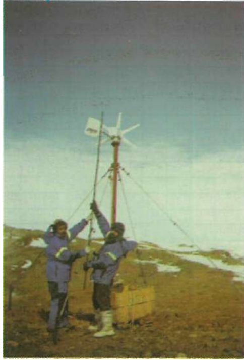
Fig. 4: Servicing wind battery charger at communication repeater station at Vettaiah peak
