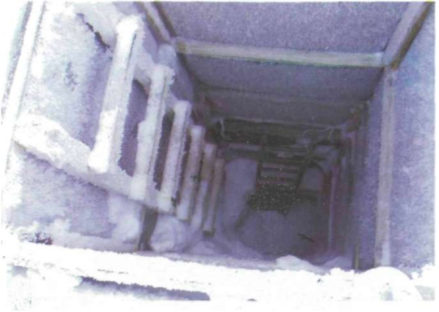
Photo-4: The entrance shaft in the roof of the buried building
