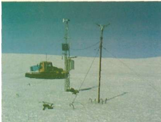
Fig. 6: The AWS with the Wind Electric Generator
