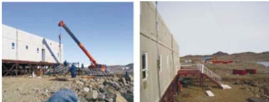
Fig. 8 : The extended platform under construction and the finished look
