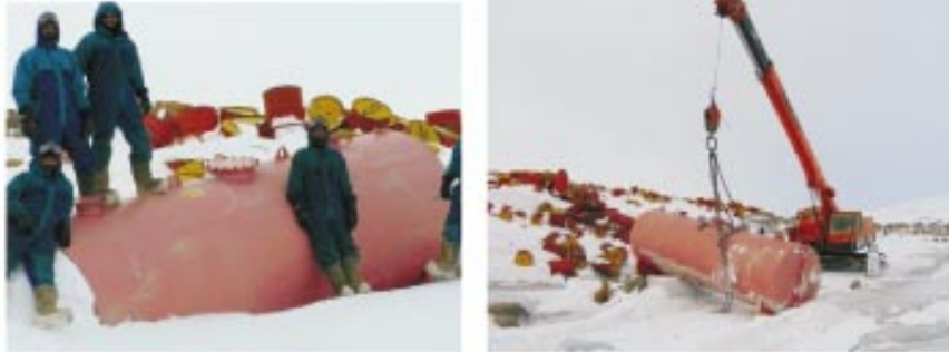
Fig. 20 : 10 KL fuel tank recovery operation
