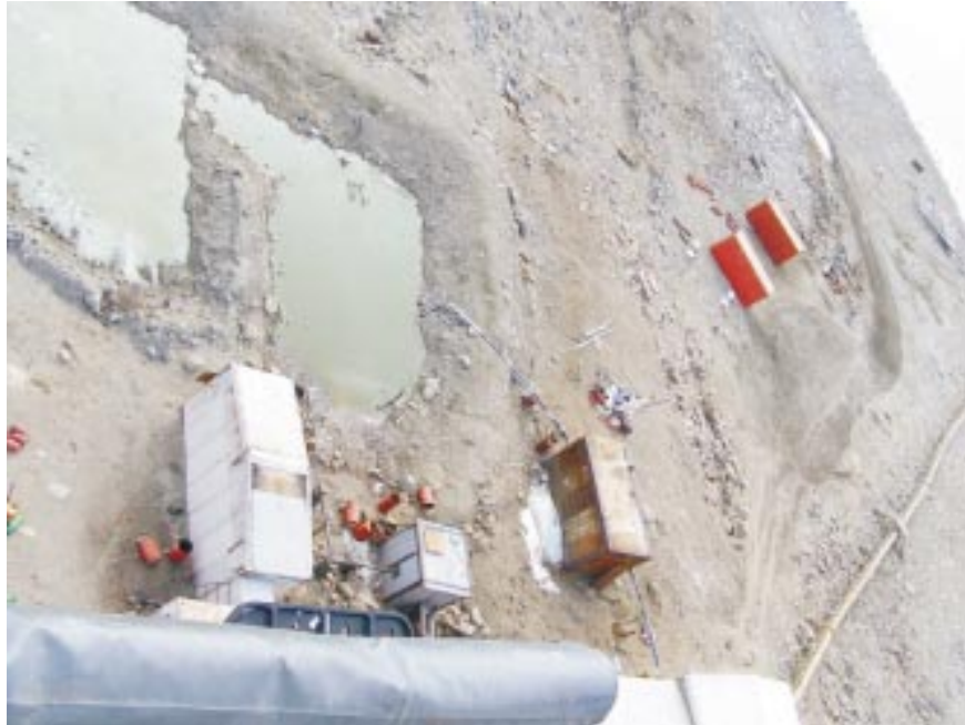
Fig. 26 : The Klargesters and soak pits
