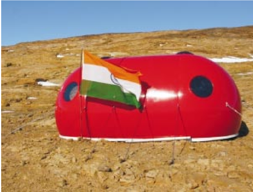
Fig. 14 : Placement of 'Melon Hut' at Larsemann Hills as the first Indian structure
