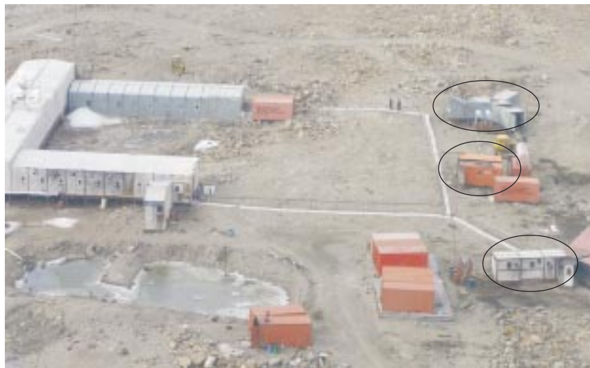
Fig. 19 : The new look of levelled rear station area, generator complex and galley route with blizzard line
