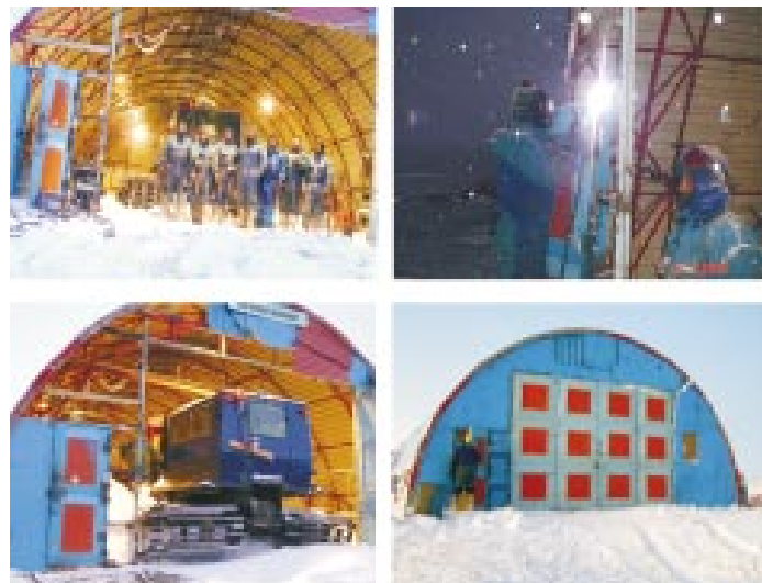
Fig. 22 : Repair work during polar nights and restoration of the workshop gate
