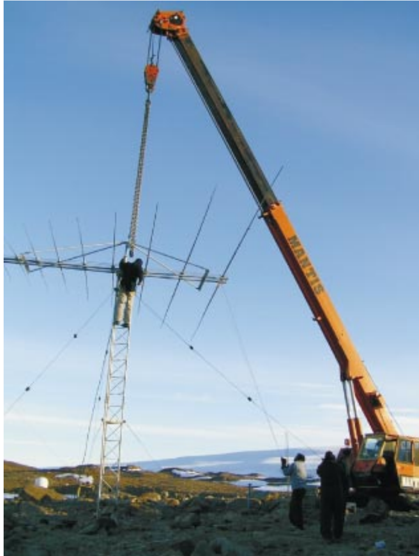
Fig. 2: Repositioning and erection of HF communication antenna
